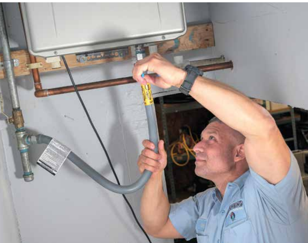
▲ Jimenez works to tighten a gas line on a Noritz tankless water heater at a residential property. A big part of the company's work is installing and repairing tankless water heaters.
