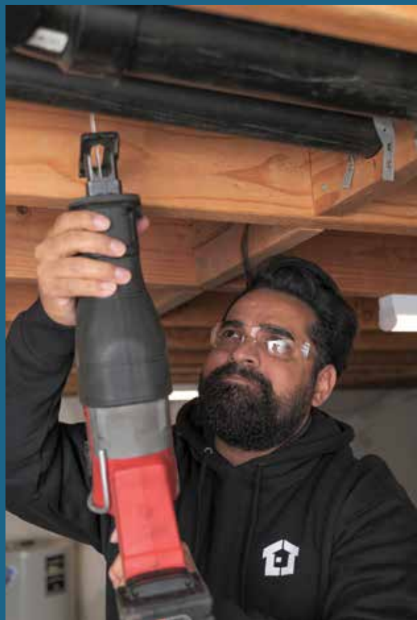
▲ Luis Sanchez, a plumber with EJ Plumbing in Santa Clara, California, gets ready to make a cut on a pipe with a Milwaukee Tool reciprocating saw.
