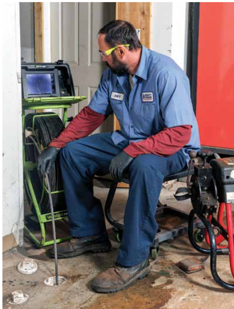
Joey Ryzoc uses an EnviroSight push camera to inspect a sewer line.
