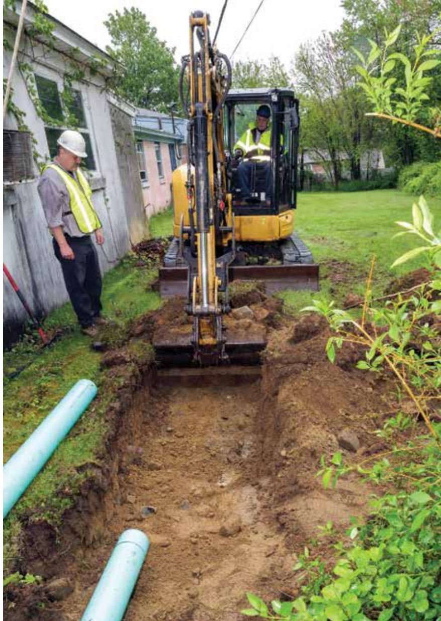
▲ Rees looks on as Peter Orsini excavates a trench in order to lay new sewer pipe.
